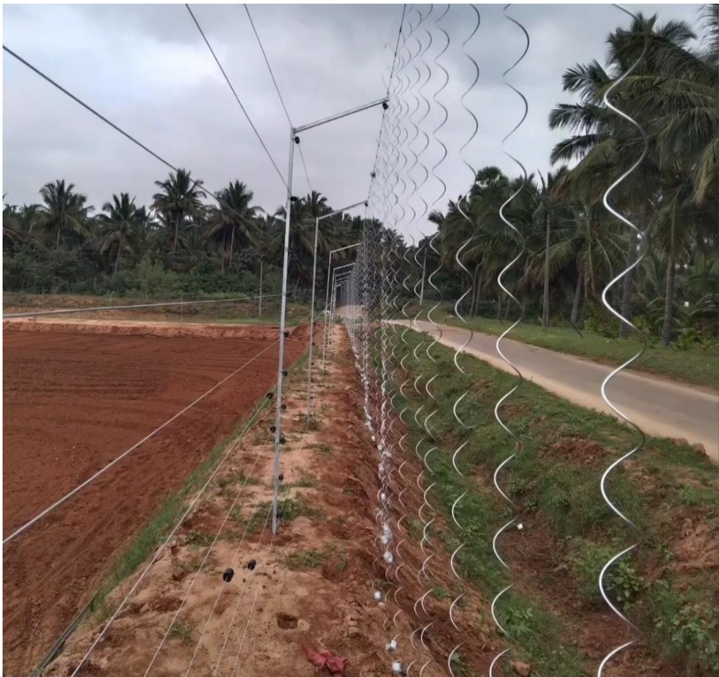
Side view of the Type 1 Hanging Fence
